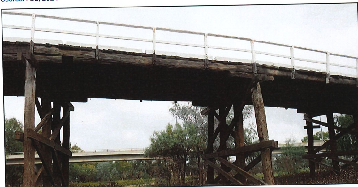
Figure 1-5: View of North Bourke Bridge timber approach girder span, looking south.
